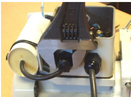
Photo 6 - Undo the cable gland to free the capacitor
