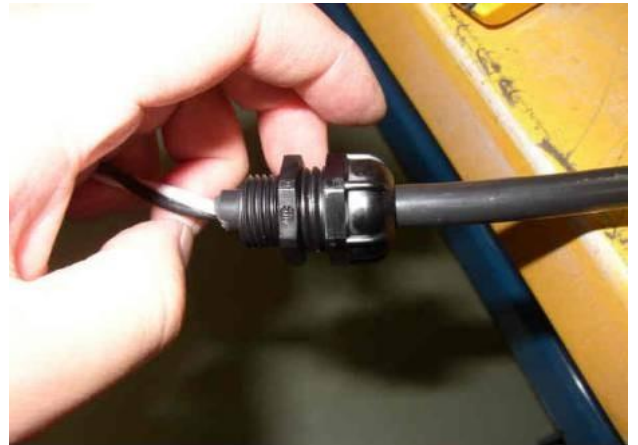
Photo 10 - Fit cable gland to capacitor lead
